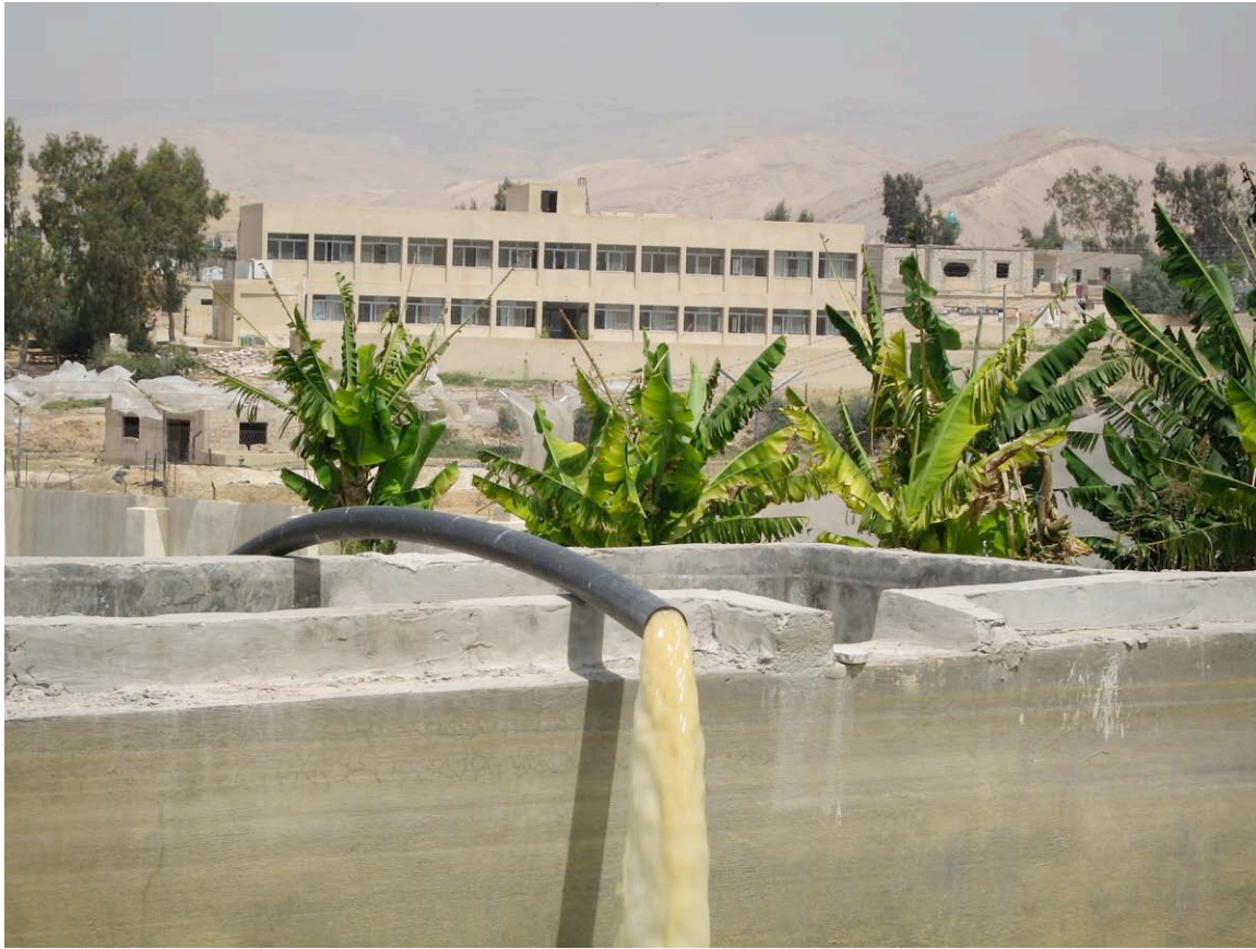
Figure 2: Well discharge in the Jordan Valley with significant sediment presenting a metering challenge.
